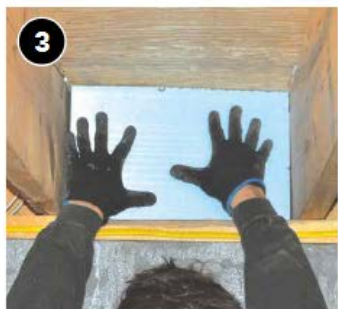
Ensure space is filled with no gaps or misalignment, and place insulation tight to rim joist.
