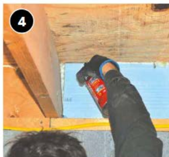
Ensure insulation is secured in place and will not move over time, then seal all of the edges with one-part foam, caulk, or mastic.
