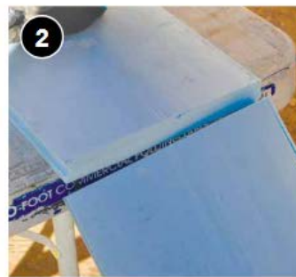
Cut insulation, either rigid foam board or wrapped/faced batts, for each individual cavity.
